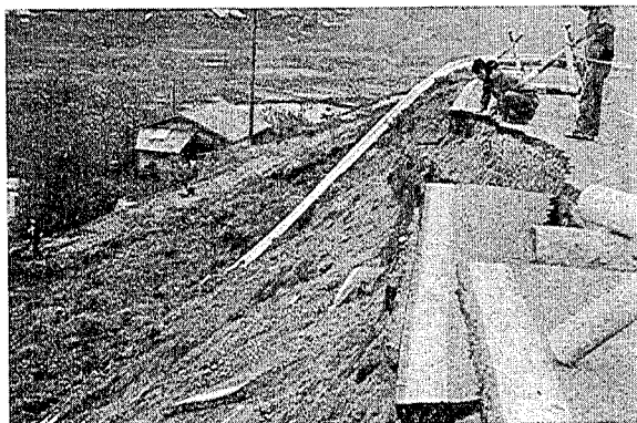
Photo 5 Slope failure of embankment at Asamizu, National Highway Route 4.
