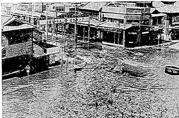
Photo 5 The inundated main street of Kamaishi City. (Courtesy of Kamaishi Civil Engineering Office) 釜石市市街部への津波浸入状況 (釜石土木事務所)
