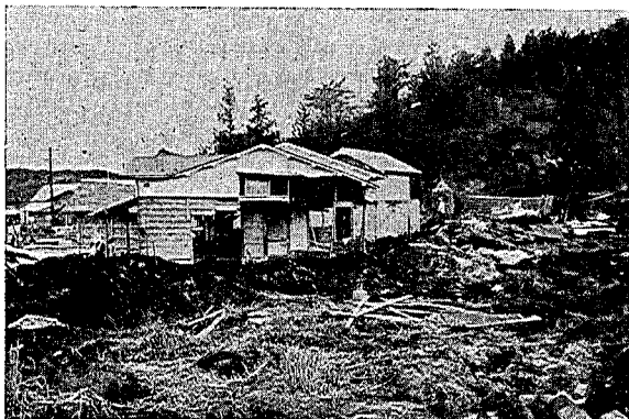
Photo 20 Damage of houses by landslide at Shitogishi area in Gonohe town. 五戸町志戸岸地区の山くずれによる家屋の被害
