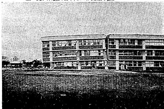
Photo 21 Damage of reinforced concrete building (Misawa commercial high school in Misawa city). Collapse in the immediate after the earthquake. 三沢商業高校校舎の被害，地震直後に陥没
