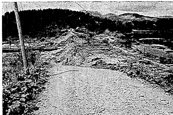
Photo 4 Damage of banking (Hayagake-numa pond in Mutsu city). むつ市「早掛沼」(締め切り堤の決壊状況)
