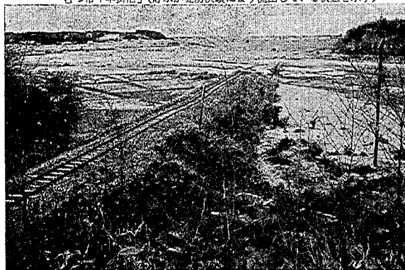
Photo 5 Damage of rice field by damage of the banking of Hayagake-numa pond. The flood by damage of the banking converted the rice field into a temporary lake (near Hayagake-numa pond). むつ市「早掛沼」の反対側の被害
