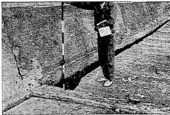
Photo 25 Cracks in the parapet wall of the coastal dike at Momoishi. 百石海岸堤防のバラベツトウォール部の被害
