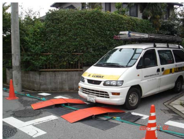
Fig. 30 A photo showing steps for a vehicle to pass over the Land Streamer
