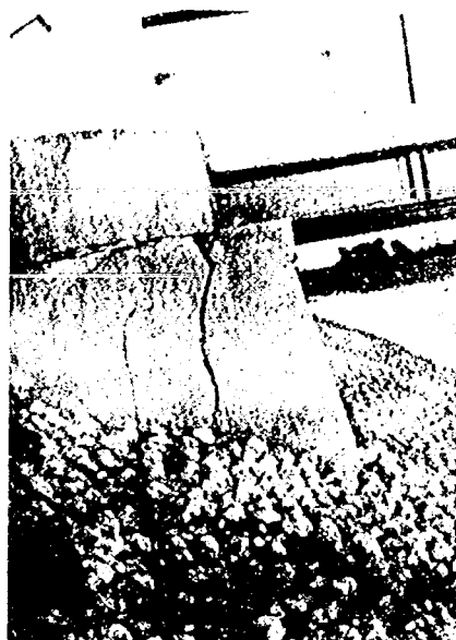
Photo. 2.18 Damage to the Takahata Bridge (3) (Damage to the Right Abutment)
