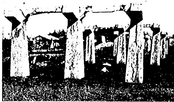
Photo. 2.12 Damage to the Piers of the Banyu Bridge (under Construction)
