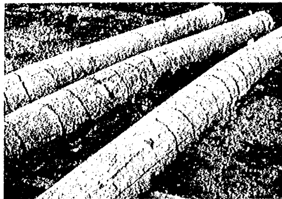
Photo. 2.57 Piles Pulled out from the Ninth Pier of the Higashi-Kosenkyo Bridge (2)
