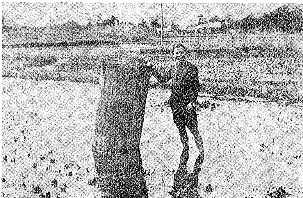
Photo. 2 Wooden piles which floated up from a rice paddy at Chigasaki during the Kanto Earthquake
