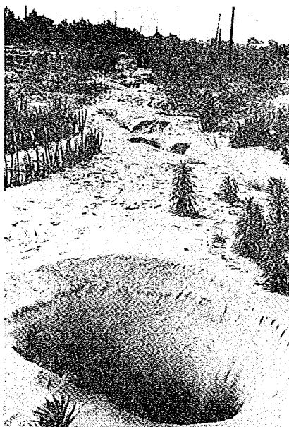
Photo. 10 Large holes in the liquefied ground at the zone 10 in Fig. 4 which is the old riverbed of the Shinano river during the Niigata Earthquake
