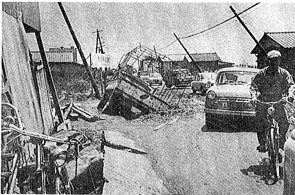
Photo. 9 A truck which sank into the liquefied low bank of the National Highway No. 7 at Ebigase during the Niigata Earthquake
