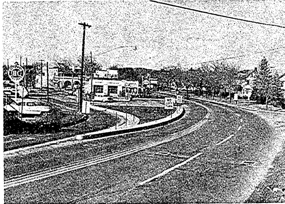
After Permanent Channelization Looking Westbound
