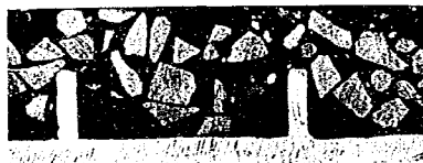
Fig. 8.7. Cross section of the wearing surface on the Duesseldorf-Neuss Bridge. Bituminous-mix between flat bars
