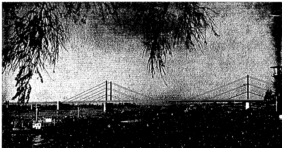
Fig. 1.16. View of Duesseldorf-North Bridge
