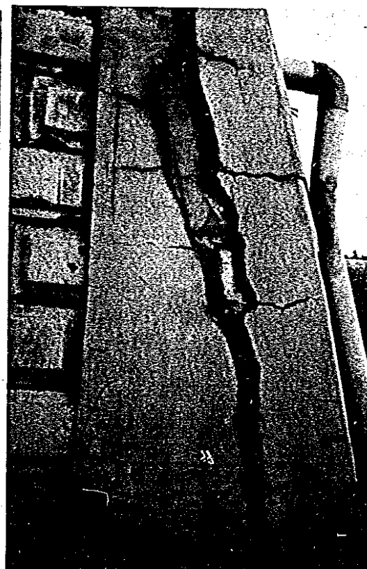
Photo-30 Damages of Sankei Hospital in Sobetsu Town.
