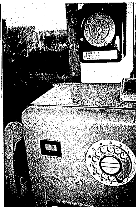
Photo-21 Damages of Telecommunication Facilities.
