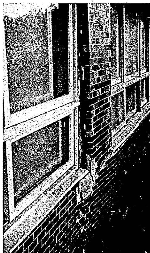
Photo-27 Damages of Sankei Hospital in Sobetsu Town.
