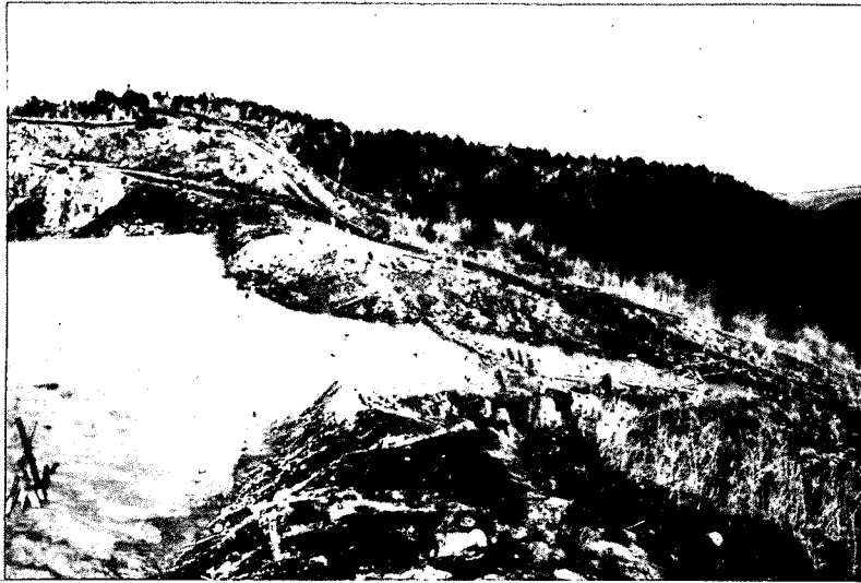
Photo 3. Flowing Out of Sludge Caused by the Failure of Dykes of its Reservoir
