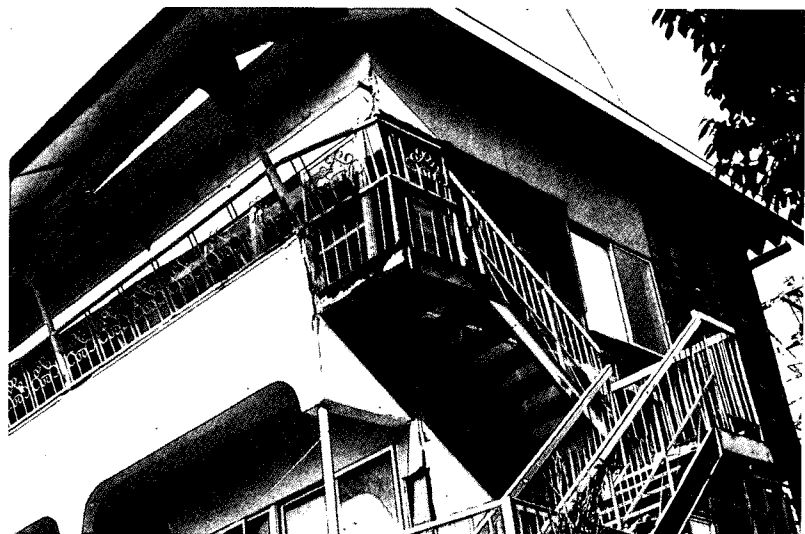
Photo 6. Residential Damage in Shimoda City
