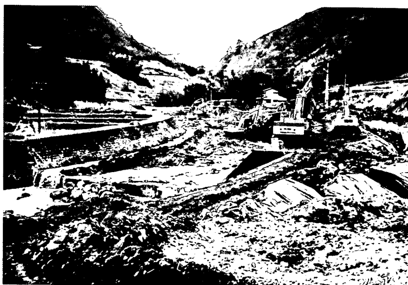
Photo 2. Sludge Removal from the Mochikoshi River
