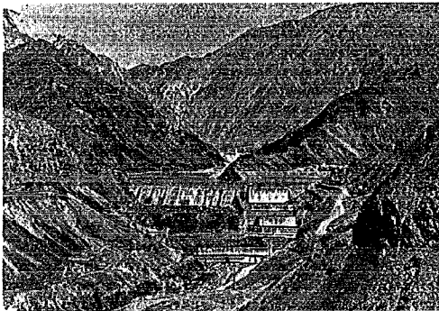
Photo 2 Devastation of Mountain Area and Ashio Dam (Watarase River).
