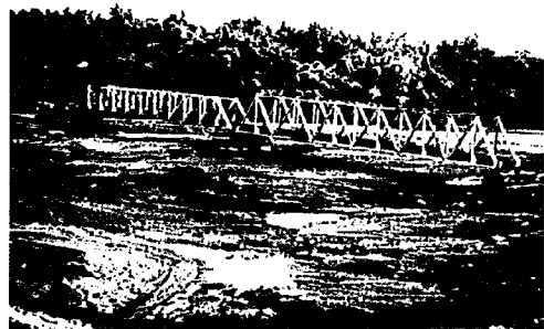
Railway bridge had collapsed by mudflow at 1975
