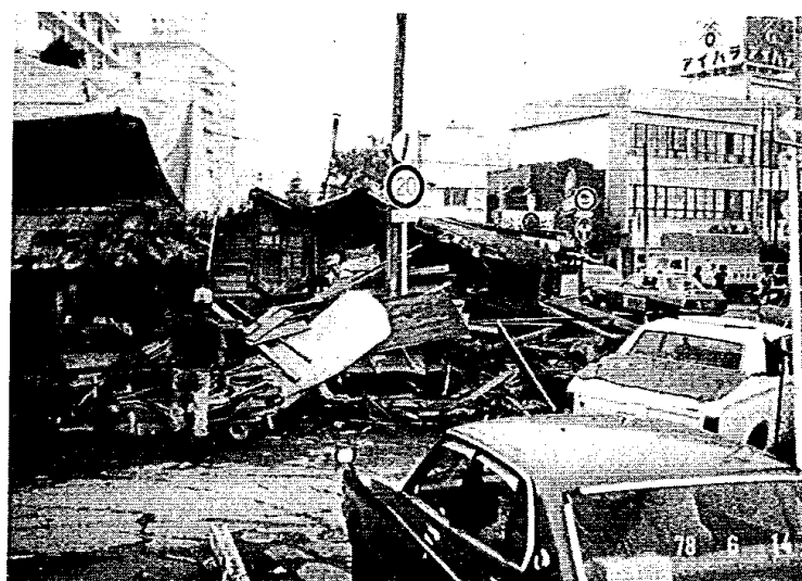
Photo. 3. Damaged Wooden House at Naga-machi, Sendai
