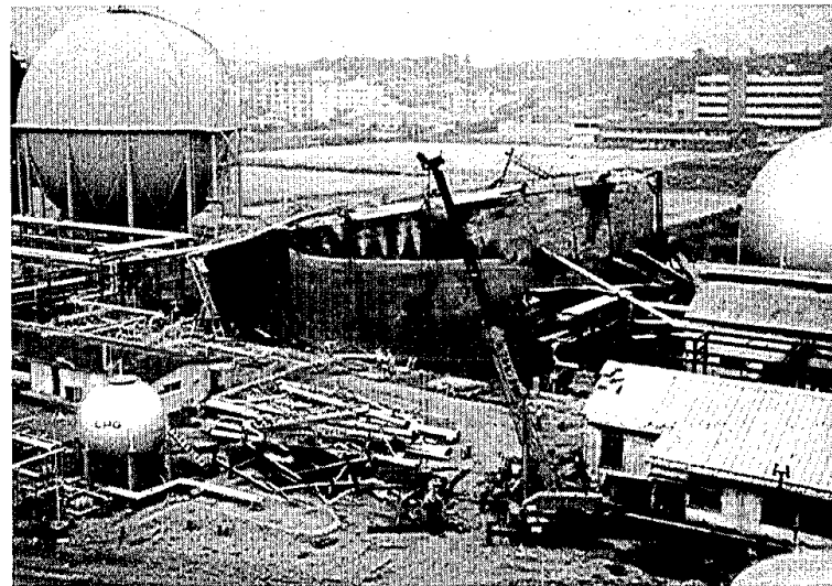
Photo. 14. Burned Gas Holder at Harano-machi, Sendai
