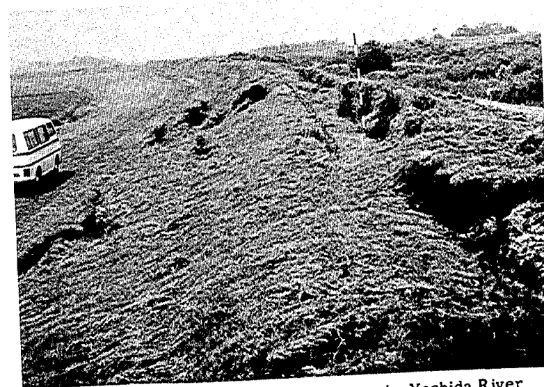
Photo. 6. Subsidence of Dyke Settlement at the Yoshida River
