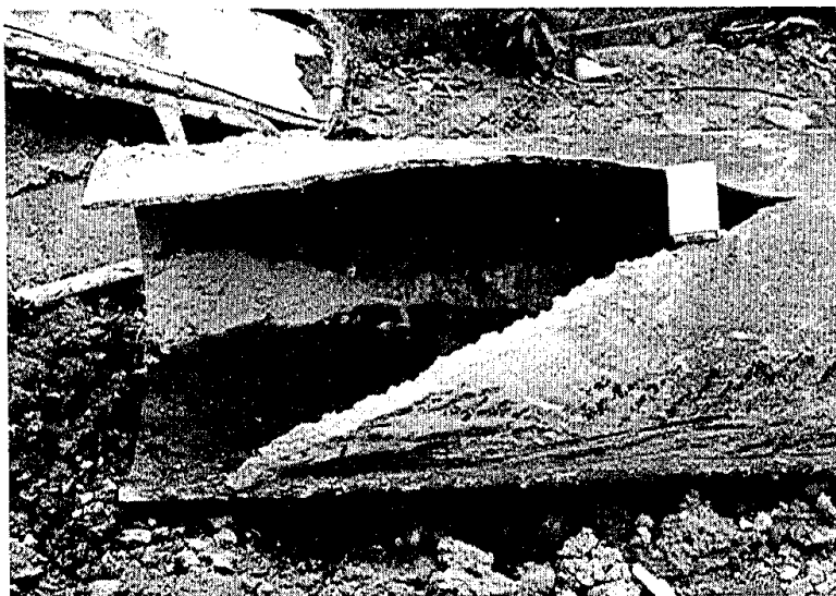
Photo. 11. Damaged Conduit of 400 mm at Mikoyama 4, Sendai
