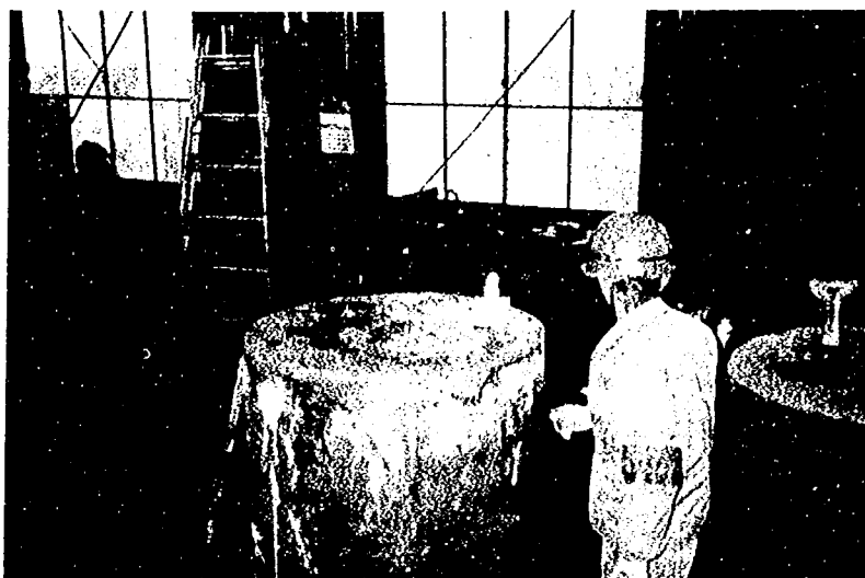
Photo-5. Mortar Casting
