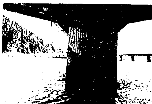
Fig. 52. Damage to Pier-4 of Shizunai Bridge
