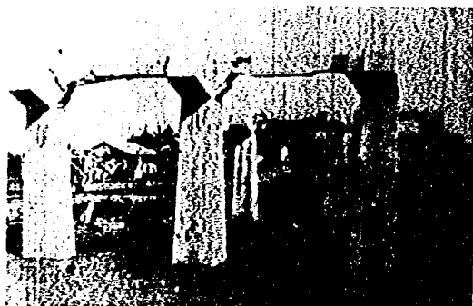
Fig. 4. Damage to the Piers of the Banyu Bridge while under Construction
