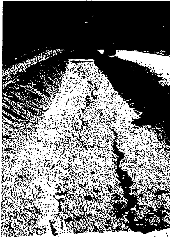
Photo 1 Cracks parallel to dam axis (Makio Dam)
