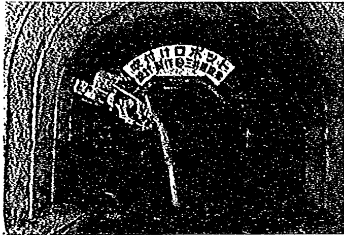
Photo 2 Spraying robot type SL-2 for small cross sections (Used for the work on the western side of the Kagosaka tunnel on the East Fuji route of the Japan Highway Public Corporation)
