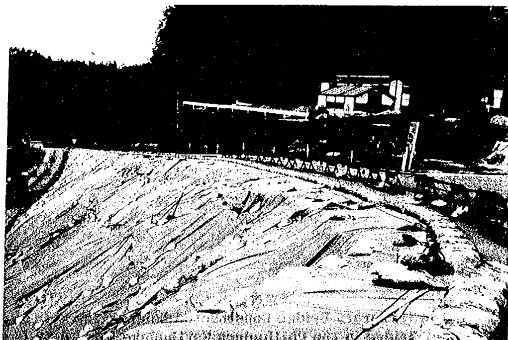
Photo. R.3.3 Surface Water Drainage Work in the 1984 Nagano-Ken-Seibu Earthquake, Japan [Ref. R.3-4]
