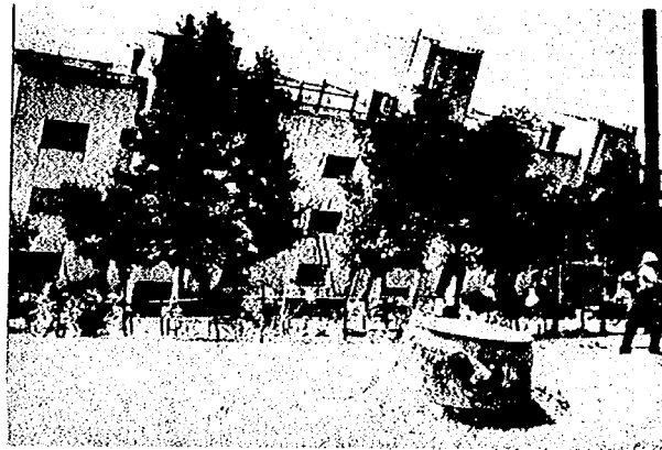
Photo. 3.11 Up-lift of Manhole and Tilting/Settlement of Building in the 1964 Niigata Earthquake [Ref. 3-1]
