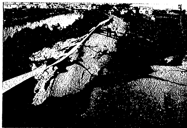
Photo. 3.6 Sliding and Settlement of Levee in the 1983 Nihon-Kai-Chubu Earthquake [Ref. 3-2]
