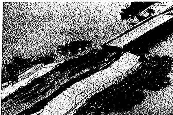
Photo. 3.2 Damage of Approach Embankment of Gomyokoh Bridge in the 1983 Nihon-Kai-Chubu Earthquake [Ref. 3-2]
