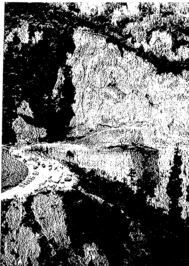
Photo. R.1.2 Large Slope Failure Occurred at the Dalton Pass of the Pan Philippines Highway [Ref. R.1-2]
