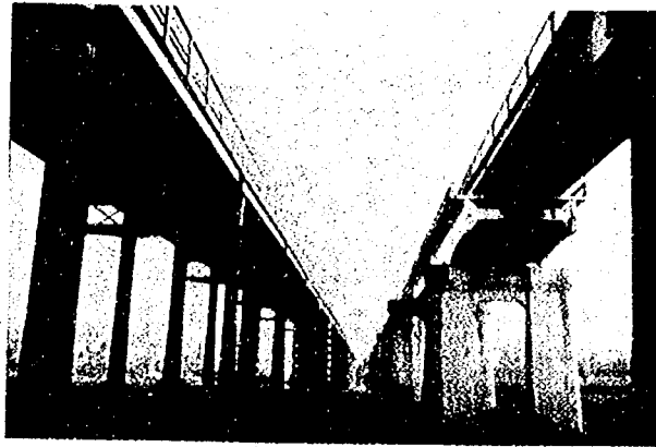
Photo. 7.4 Temporary Girder (Right-side) and Temporary Bridge (Left-side) Constructed at the Kinnoh Bridge Damaged in the 1978 Miyagi-Ken-Oki Earthquake, Japan
