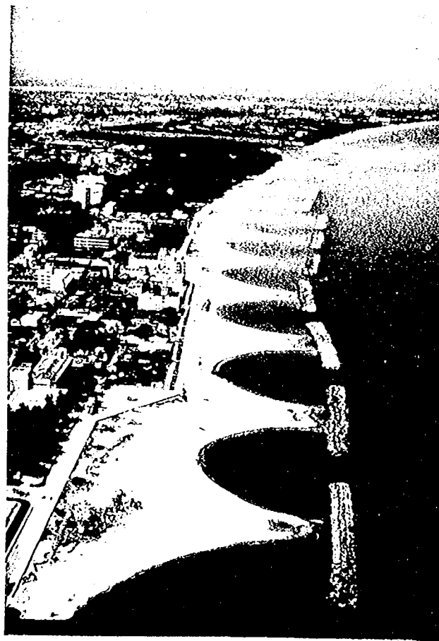
Fig. 3-1-21 Kaike Beach (after the completion of detached breakwaters).
