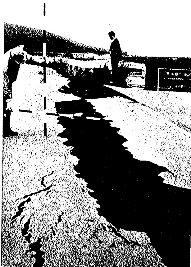
Fig. 3-1-30 Miyagi Offshore Earthquake.
