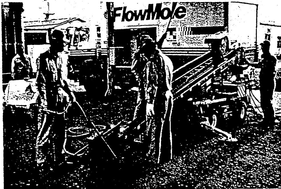
DEMONSTRATION OF TRENCHLESS TECHNOLOGY AT THE TOKYO GAS RESEARCH INSTITUTE, 10/92
