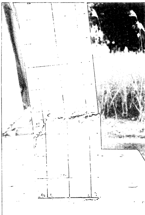
写真-4-6-6 e 1-8 供試体擁壁西面下側 (2.5m, 2回目)
