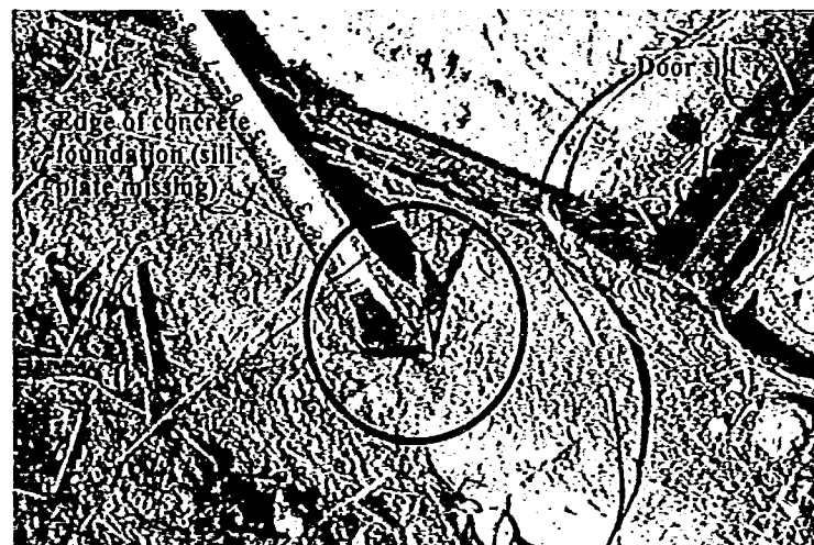
Figure 4. Evidence of nail that was used for connecting sill plate to concrete foundation.
