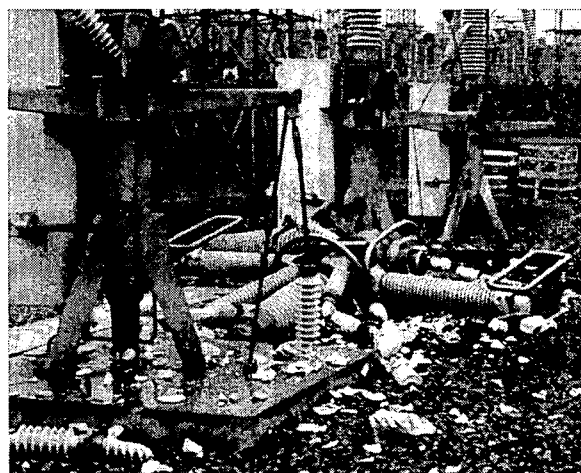
Photo. 2 Damage of Power Plant
