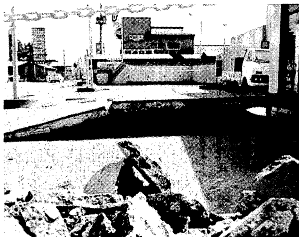
Photo. 3 Up-lift of Underground Gas Storage Tank
