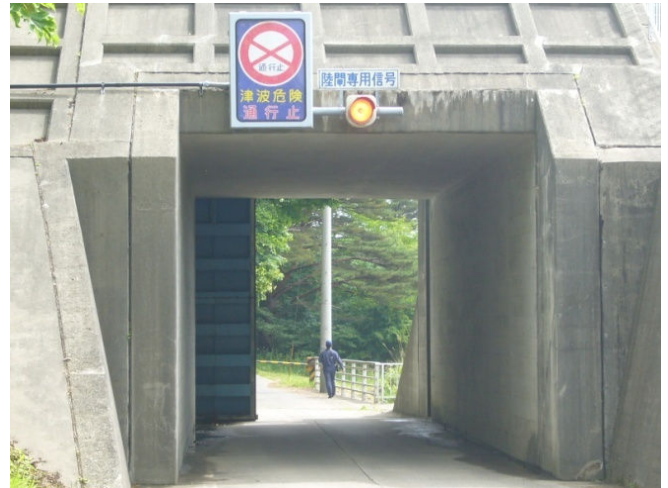
Photo3-2-2 Demonstration of the gate closing
