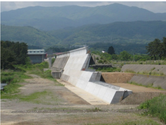
Photo3-2-3 Tsunami embankment being built in Noda village
