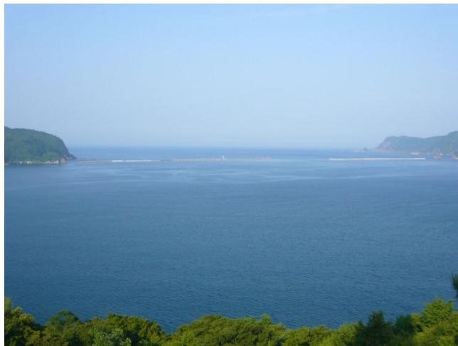
Photo3-2-9 Tsunami breakwaters in Kamaishi
