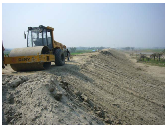
Photo 6-38 Levee under construction
