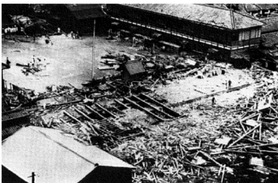
Elementary school in Osaka damaged by the Muroto Typhoon (1934) [18]
