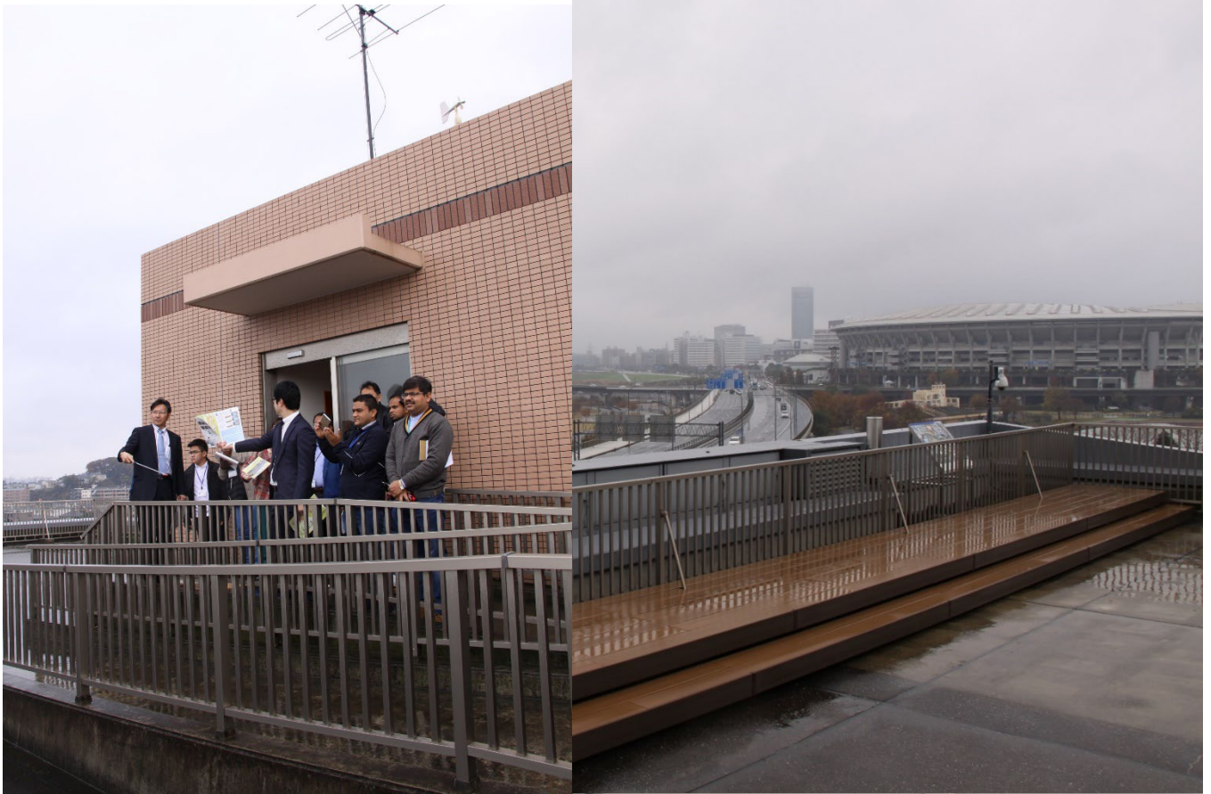
Tsurumi River Basin Center (December 5)
