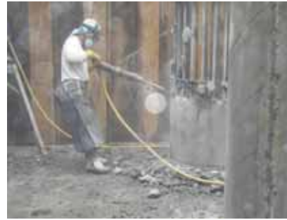
d) 杭破碎 (はつり)
