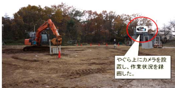
Fig.C-8 Installation of work for the camera
