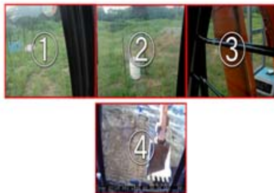
Fig.D-9 Working viewing field of the operator operating at the cabin
