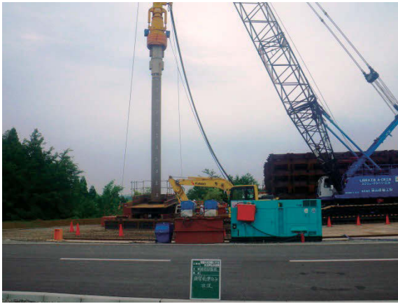
(c) 杭建込み
