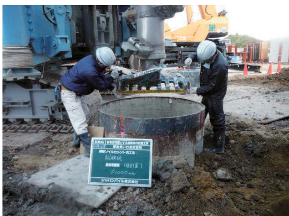
(a) 掘削径確認
