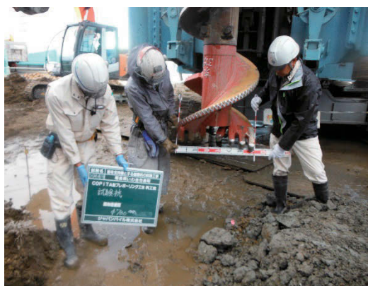
(a) 掘削径確認
