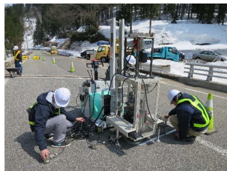
写真-1 衝撃荷重載荷試験機 SIVE (SIVE : Self-propelled Impact Vibration Equipment)
