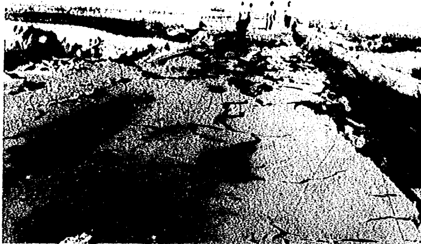
Fig. 32 Excessive Settlement of Approach Bank to Gomyoko Bridge
