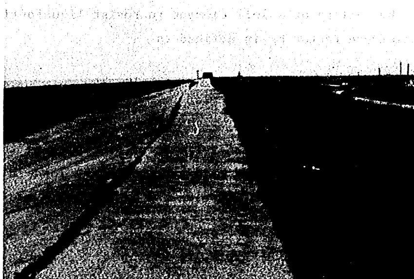
Fig. 38 Another View of Damage to Dike of Hachirogata Lagoon
