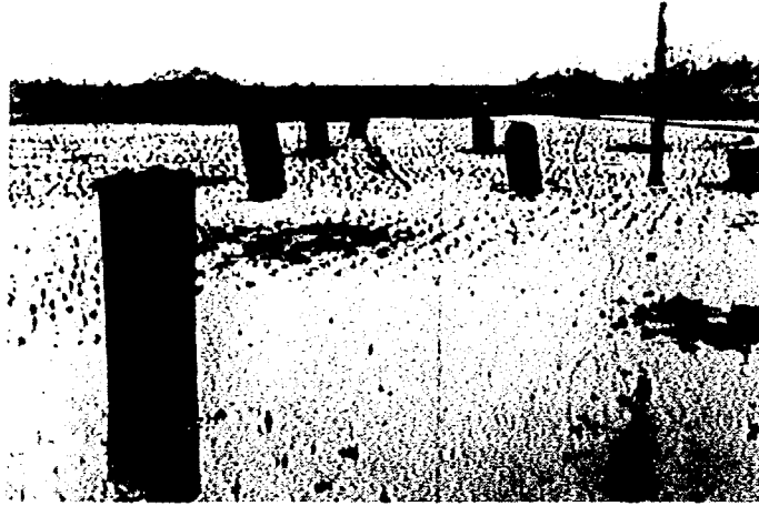
Fig. 12 Wooden Piles which Floated up from Rice Paddy at Chigasaki, Kanagawa Prefecture during the Kanto Earthquake of 1923
