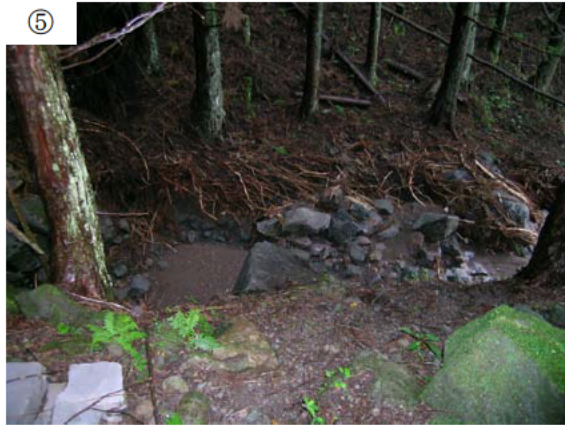
⑤ 岳本川砂防堰堤下流
