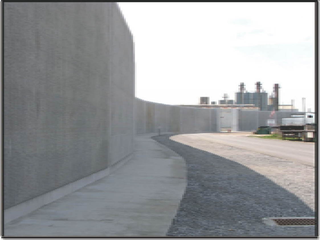
Figure 3 Floodwall at Harvey Canal
