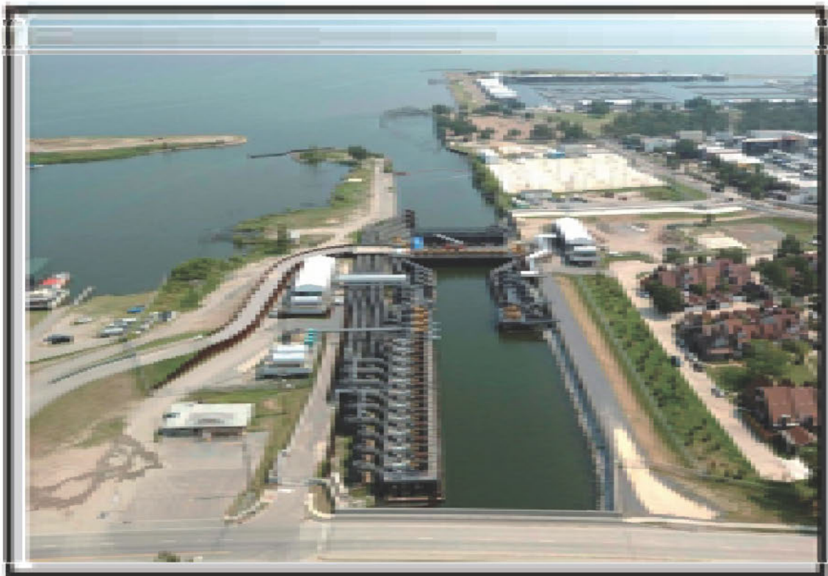
Figure 4 17 th Street Outfall Canal
