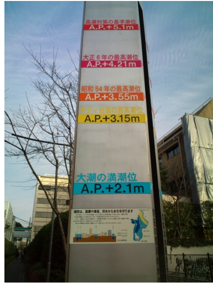
Ara River Water Level Tower
