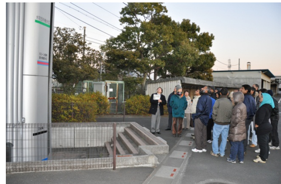
Tone River Water Level Tower
