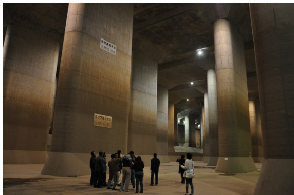
Surge tank of the Discharge Channel
