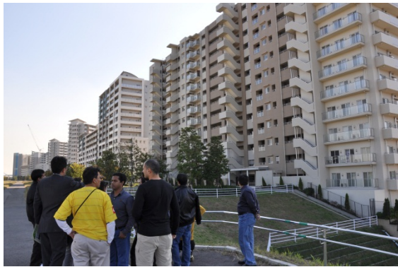
Super levee at Shinden
