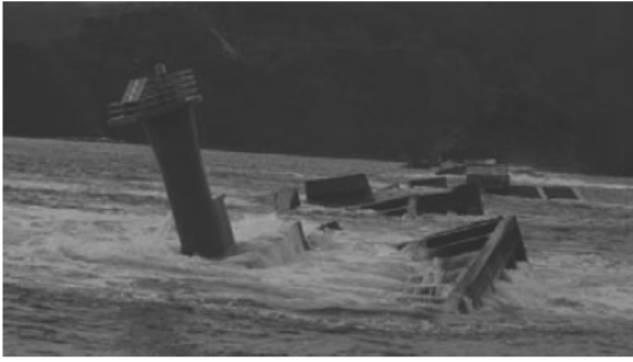
Fig. 9 Damaged offshore breakwater in Kamaishi Port
