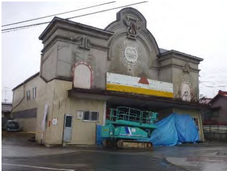
Photo 3.3 Large-scale Wood Building renovated to a Factory
