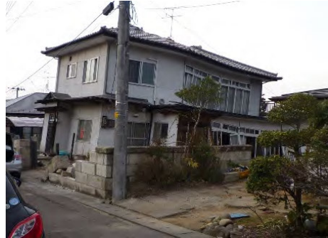
Photo 3.10 Damage of House caused by the Ground Transformation (Oritate)
