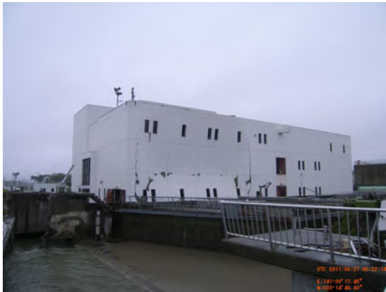
Figure 5 Minami Gamou Wastewater Treatment Plant Building.
