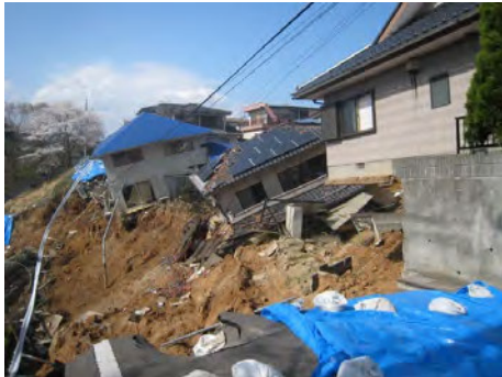
Photo 3.69 Land Sliding on Slope on the Southwest of the Hill and Sliding House
