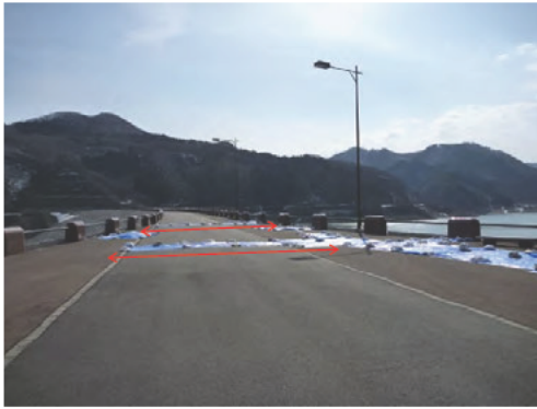
(a) Overview of the crest
