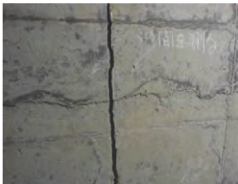
(a) Contraction joint 2J3
