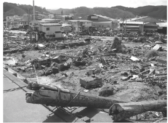
Fig. 11 Destruction of residential area behind protection dike
