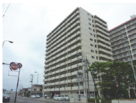
Photo 3.72 Overview of SI building B
