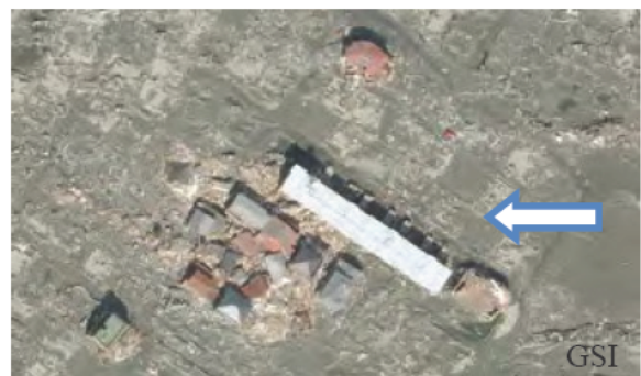
Photo 4.14 Remaining Wood Houses Behind Remaining Building
