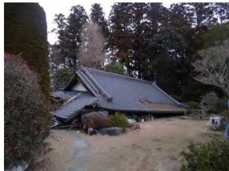
Photo 3.16 Collapsed Wood House
