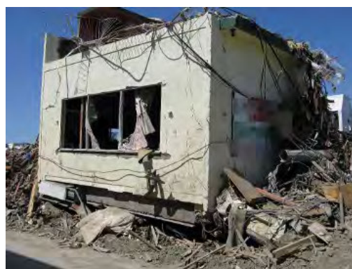
Photo 4.1 Story Collapse of 2-story Reinforced Concrete Building
