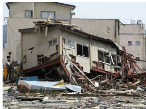
Photo 4.10 Story Collapse of First Floor in 2-story Steel Building
