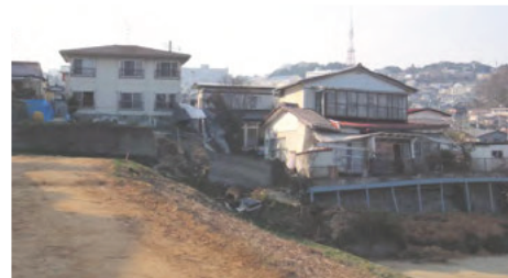
Photo 3.68 Group of Houses damaged by Sliding and Ground Transformation
