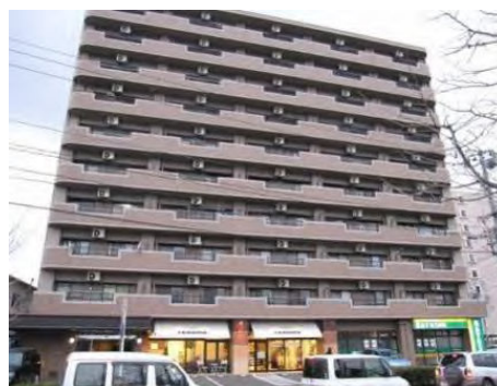
Photo 3.40 Appearance of Damaged Building
