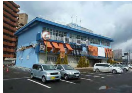
Photo 3.23 Mid-story Collapsed Building
