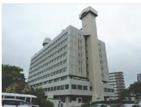
Photo 3.70 Overview of SI Building A
