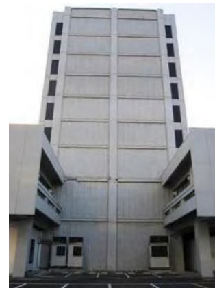
Photo 3.28 Appearance of Damaged Building
