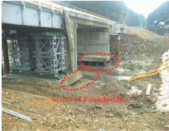
Fig.6(3) Nijyuichihama Br. (April 9, provided from Tohoku Regional Development Bureau, MLIT)
