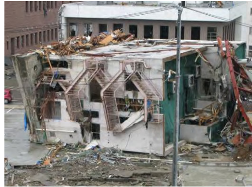
Photo 4.9 Overturning of 3-story Steel Building
