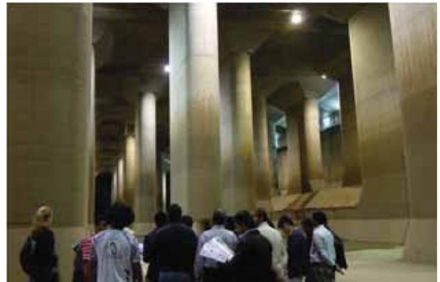
Surge chamber in Metropolitan Area Outer Underground Discharge Channel
