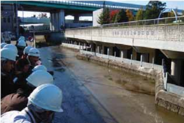
Intakes of holding ponds below Bikuni Bridge, Shirako River
