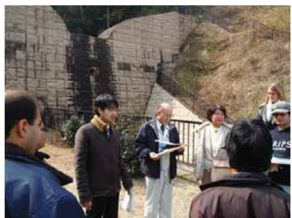
Erosion control weir in Hiroshima
