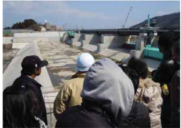
Hii River Diversion Channel construction site
