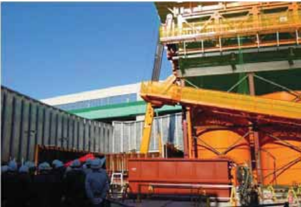
Shaft construction site
