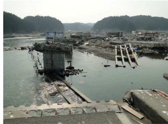
(a) Collapse of bridge due to land slide (b) Collapse of bridge due to tsunami Figure 8 Collapse of bridge caused by effect that are not mainly affected by ground shaking
