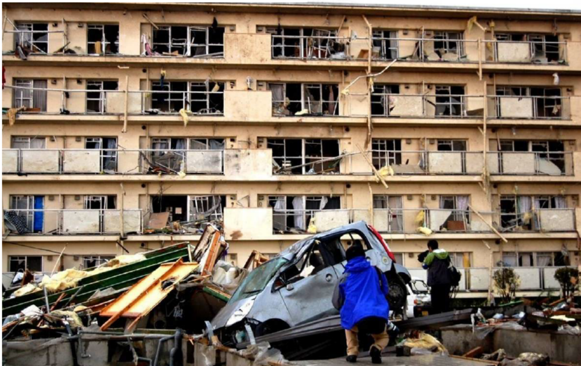
Photo 18 Damage to a 5-story apartment building
