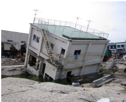
Fig. 12 Tilting by scouring
