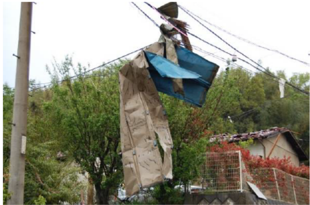
Photo 15 Metal roofing hung on power lines
