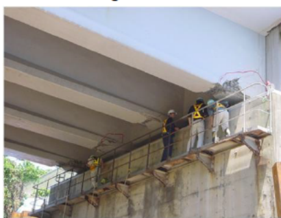
Figure 2 Walkway for Inspection
