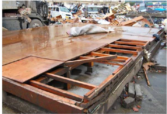
Photo 6 View of the 1st story floor of the structure in Photo 7
