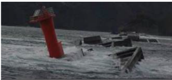
Photo 3.1 Damaged North Breakwater in Kamaishi Port
