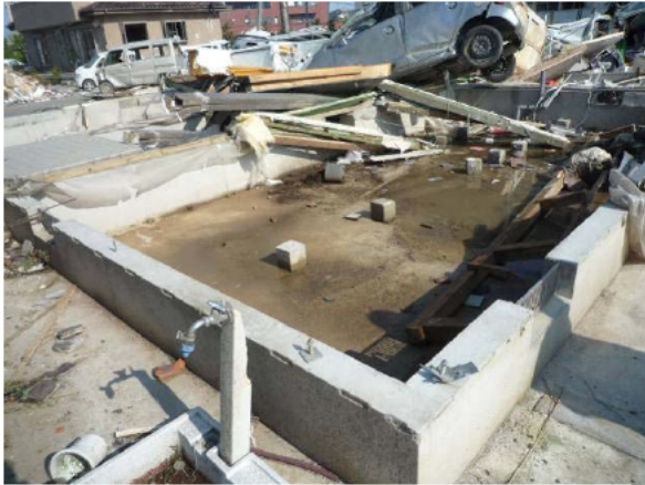
Photo 5 Foundation (corner section) of the structure in Photo 7
