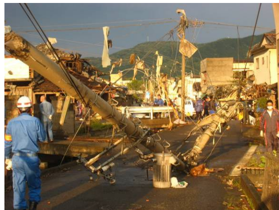
Photo 22 Broken and tilting utility poles
