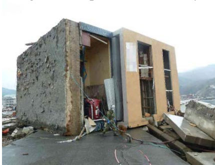
Fig. 11 Overturning
