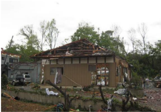
Photo 10 A damaged hip roof
