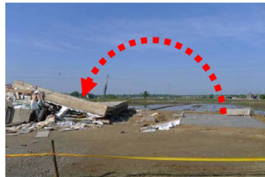
Photo 2 Relation between the building's position and the position of the overturned section
