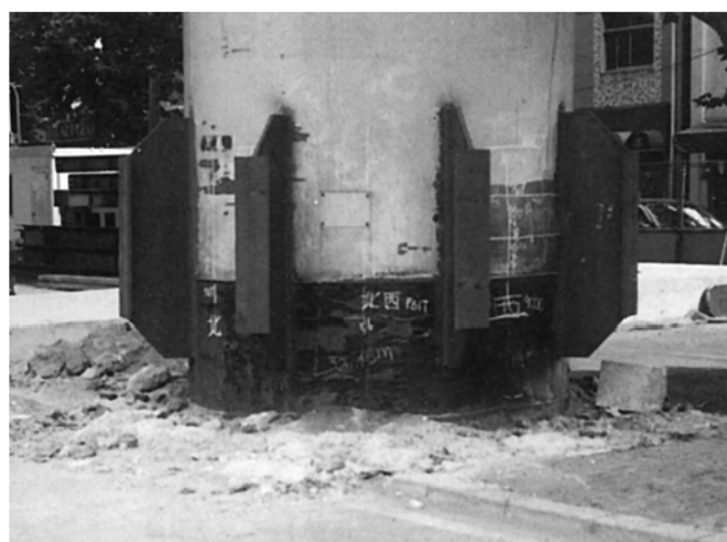
Photo 3.4.3 Emergency Measure for Buckling Section of Steel Piers
