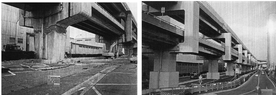
(a) Before Restoration
