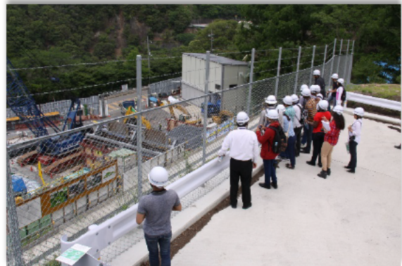
Construction site of Amagase Dam Reconstruction Project
