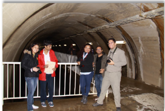
Sagurigawa Dam, MLIT
