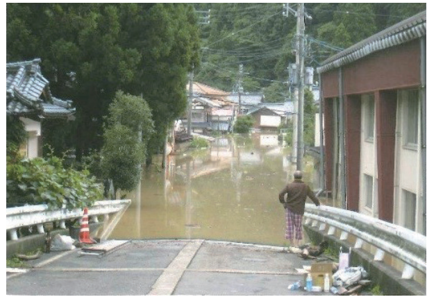
Photo 2-3-1 Flood damage in Aga Town (July 30, 2011)
