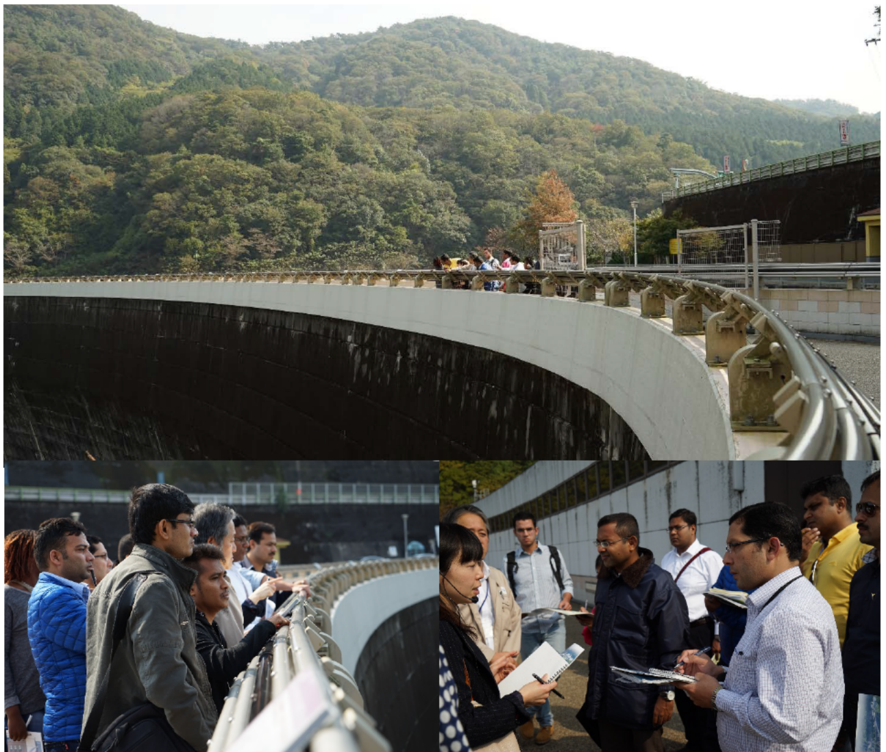
Amagase Dam, (October, 30)
