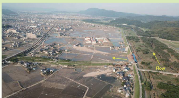
Flood damage in Mabi Town due to a levee breach along the Oda River
