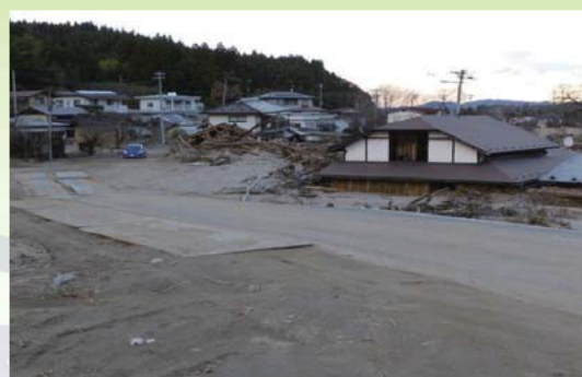
A house half-buried after a flood with a massive amount of sediment hit the area (Marumori Town, Miyagi Prefecture)
